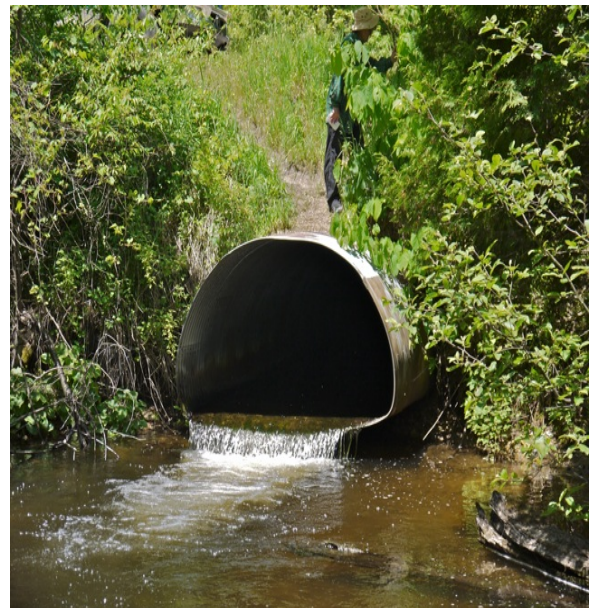
Perched outlet creating fish passage barrier
