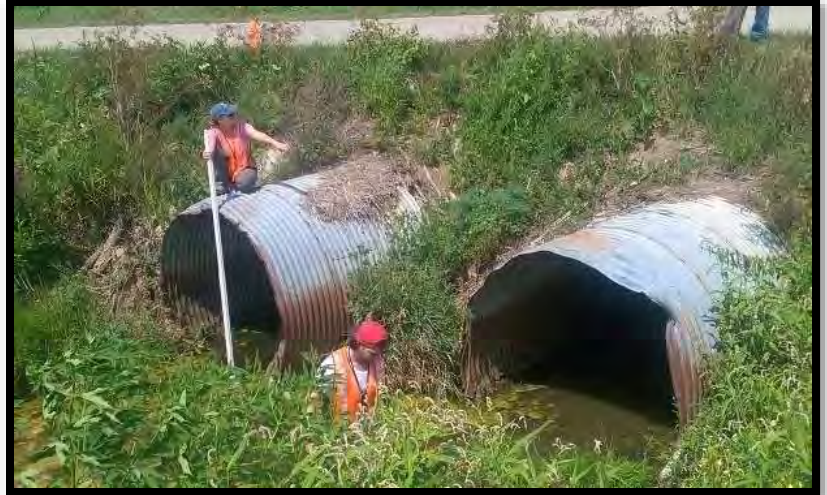
South Branch Macatawa River: Measuring culverts and water depth
