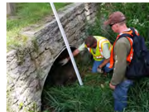
Inspecting a culvert in Park Twp.
